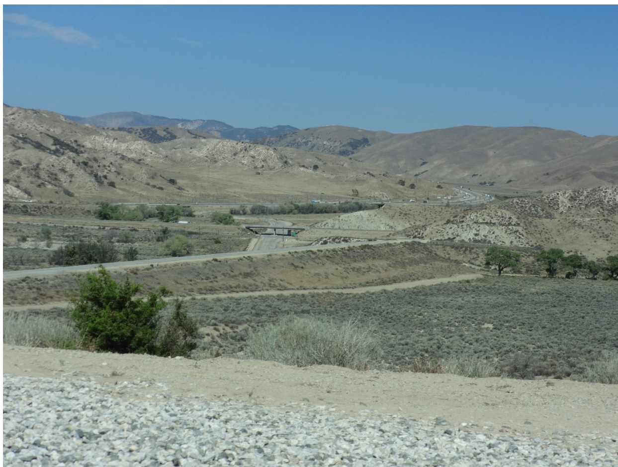
Figure 3.3-2. Quail Detention Embankment, Looking Northwest from the Peace Valley Pipeline Intake Embankment
