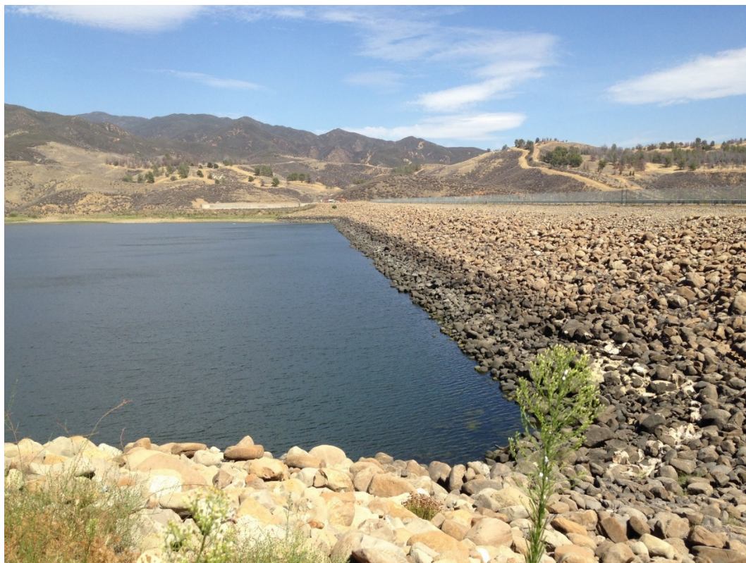
Figure 3.2-5. Elderberry Forebay Dam and Elderberry Forebay Looking East
