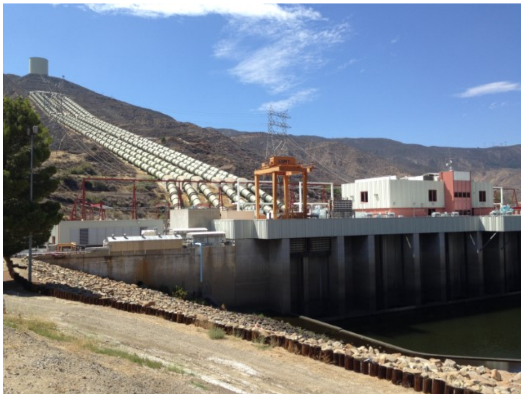
Figure 3.2-4. Castaic Powerplant and Penstocks from the East Looking West
