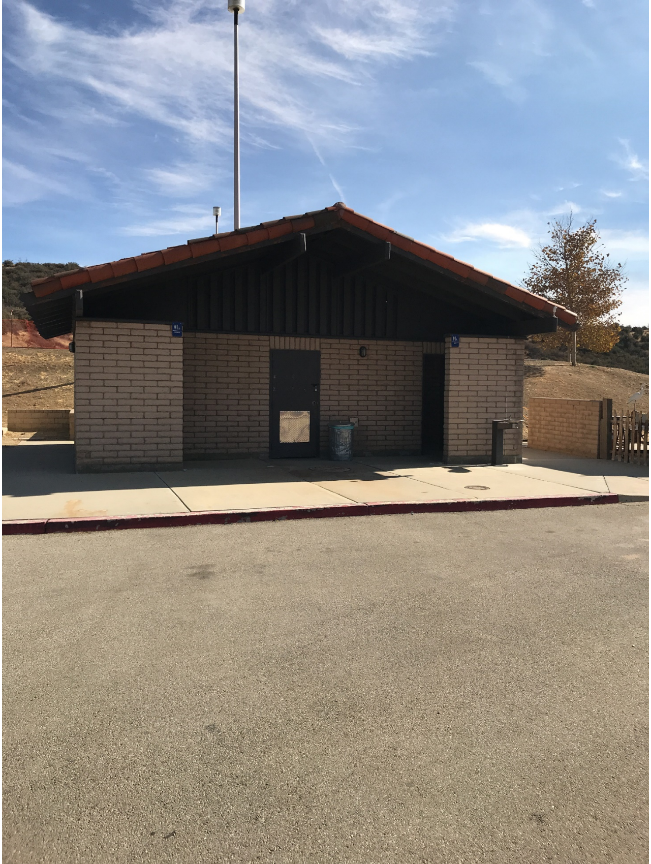
A3034R1 Vaquero Restroom Service Basic National Forest (FS) 240 1997
