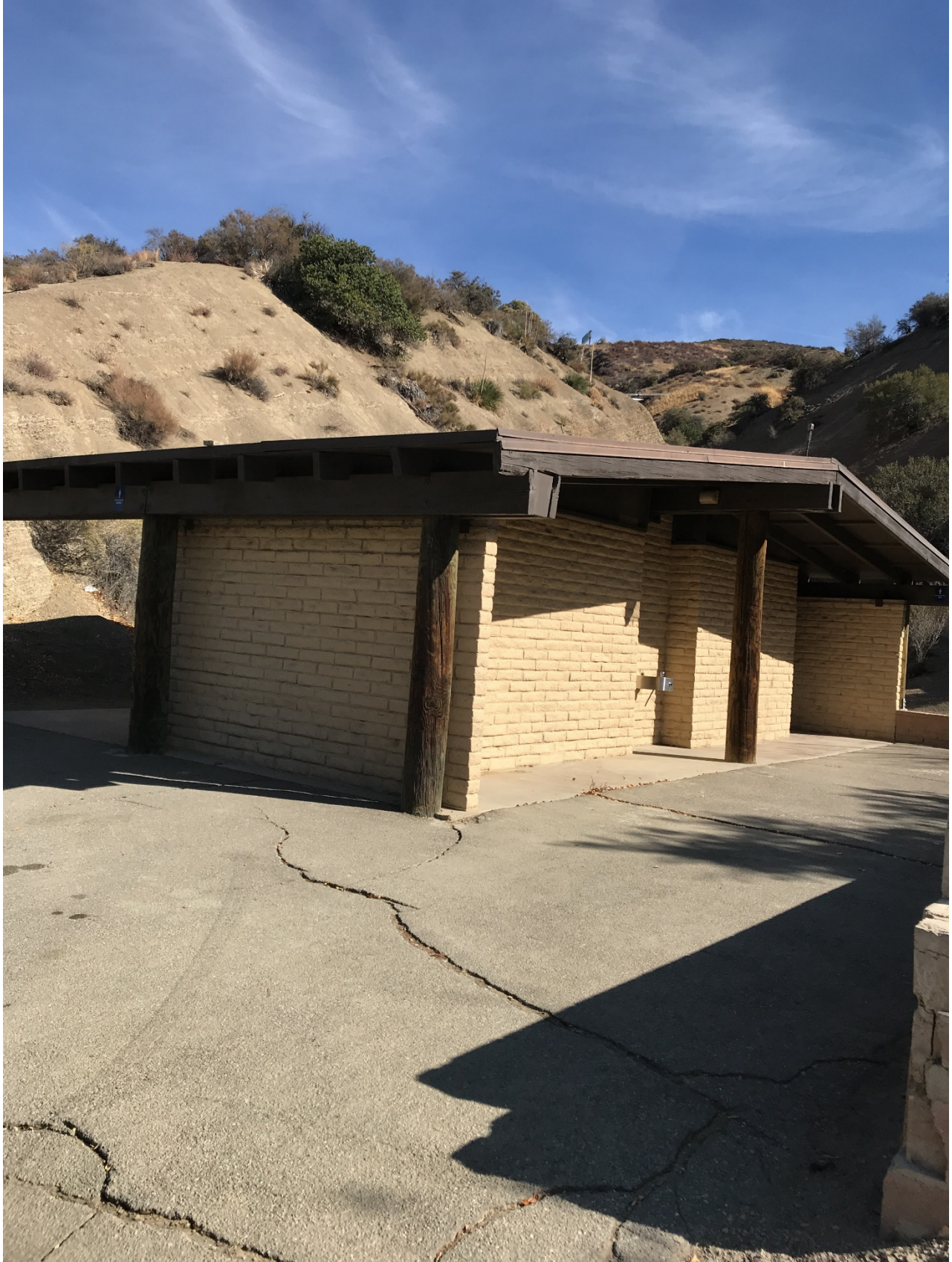
A3019R7 Emigrant Landing Restroom 7 Service Complex National Forest (FS)
