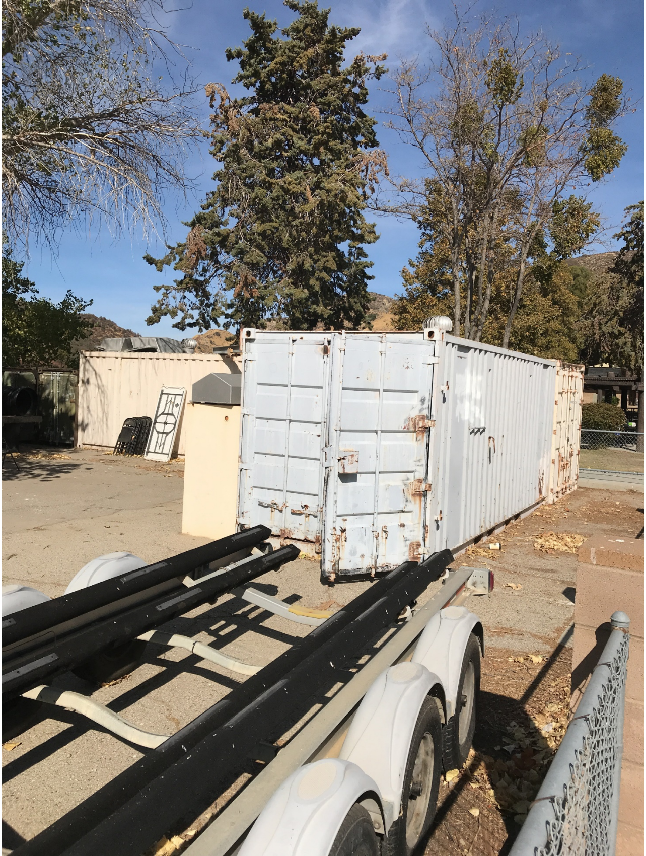
A3019ST 1 Emigrant Landing Storage Building 1 Storage Basic National Forest (FS) 190 1984
