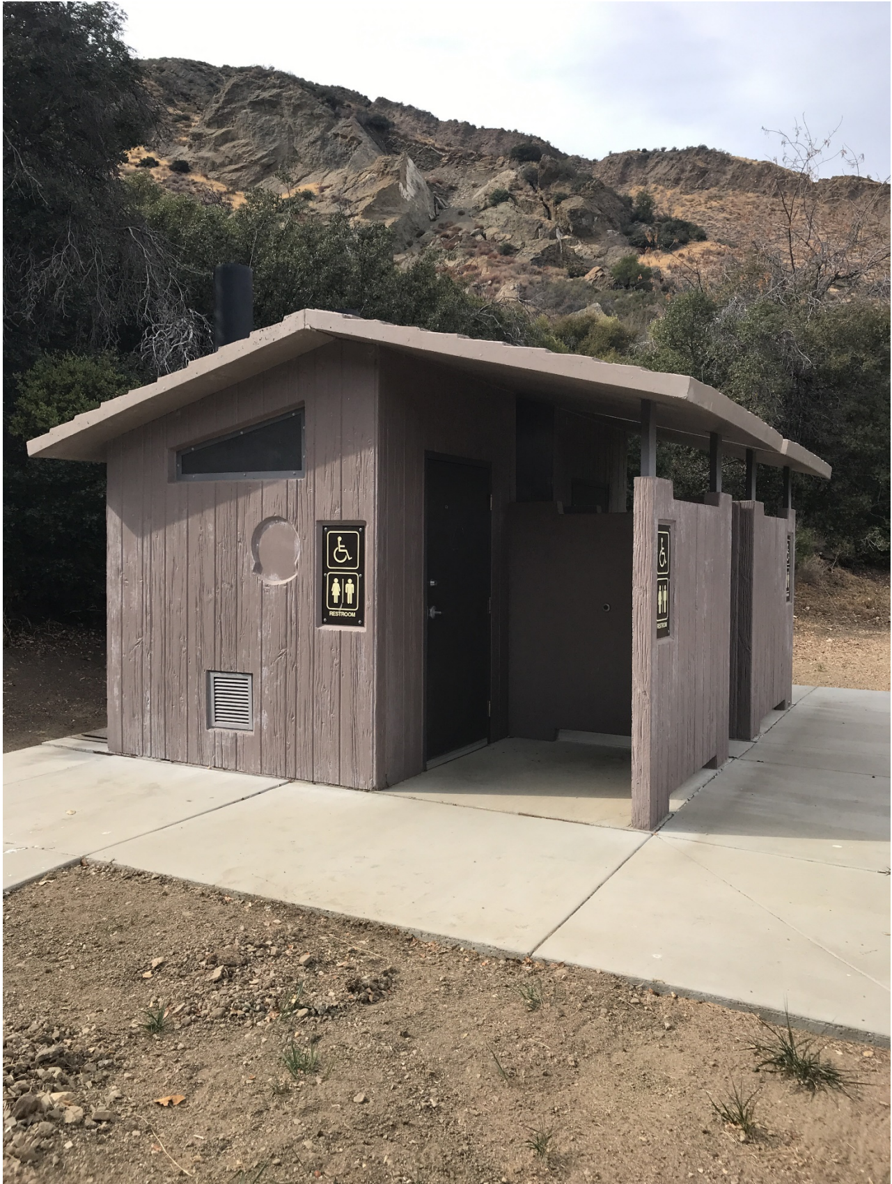
Building A3017R: Bear Trap Boat-In Site Restroom, approx. 55sq. ft, built in 1974, and photo taken from Northwest corner
