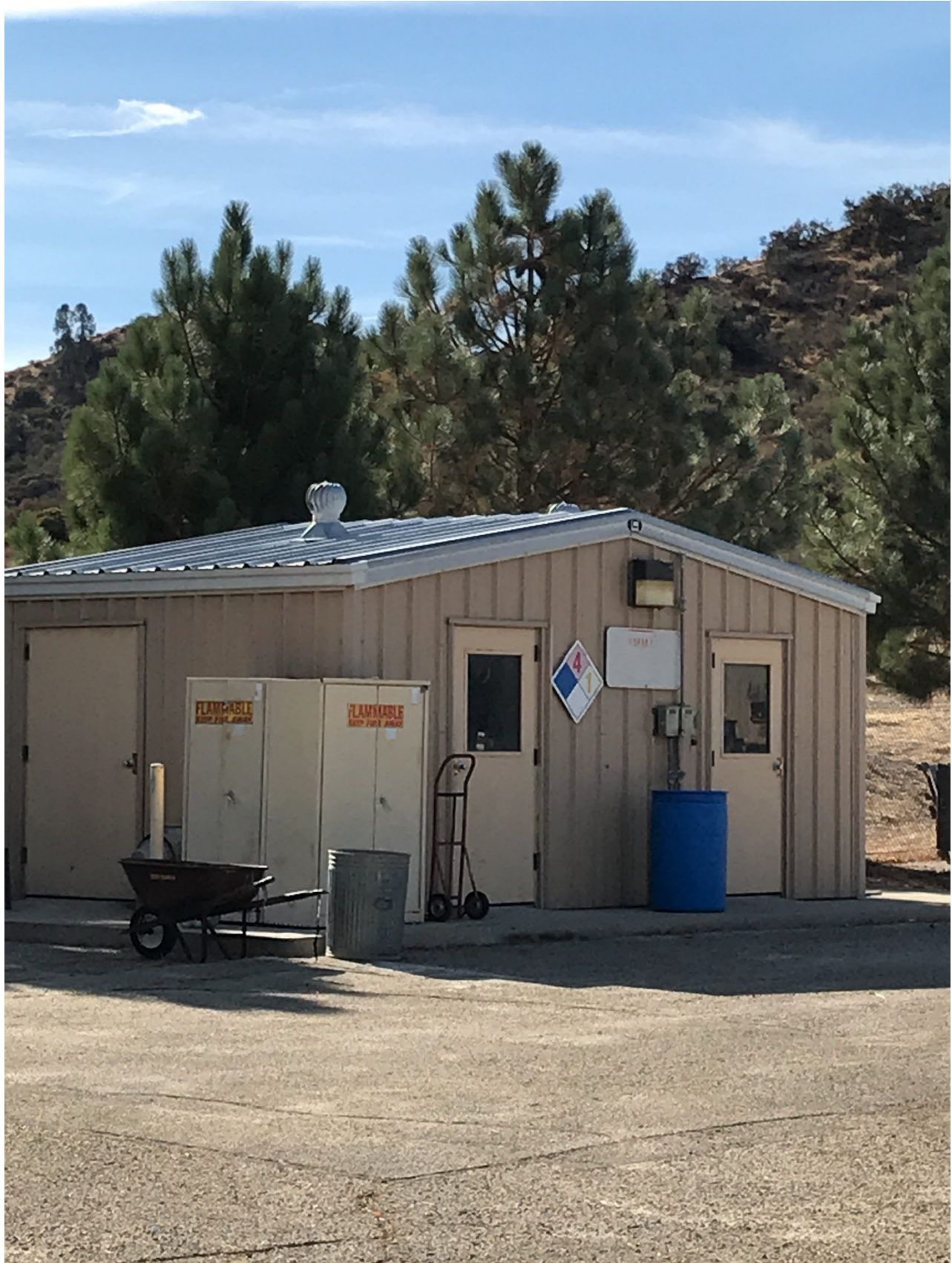
2523 Los Alamos Gas House Storage Complex National Forest (FS) 240 1983
