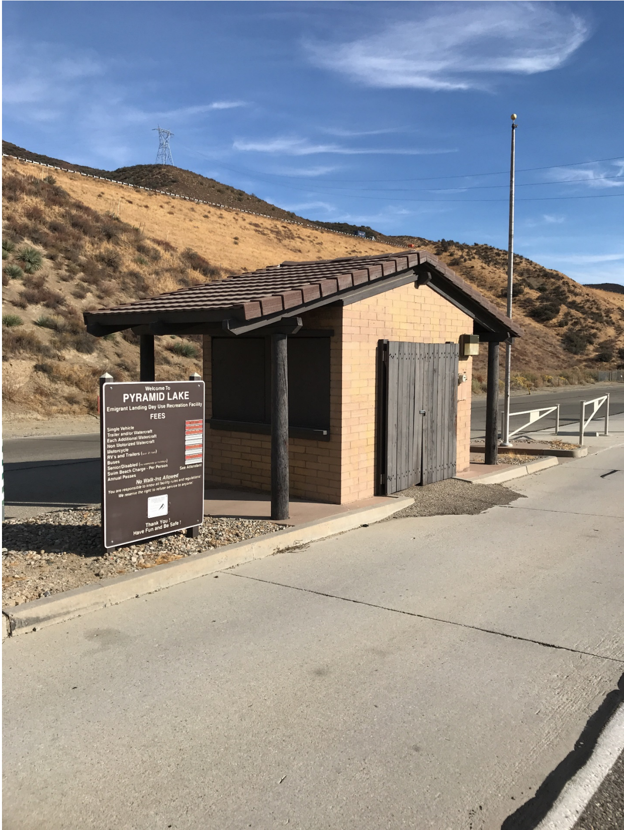
Building A3019ES: Emigrant Landing Entrance Station, Approx. 267sq. ft, built in 1984, and photo taken from North West corner
