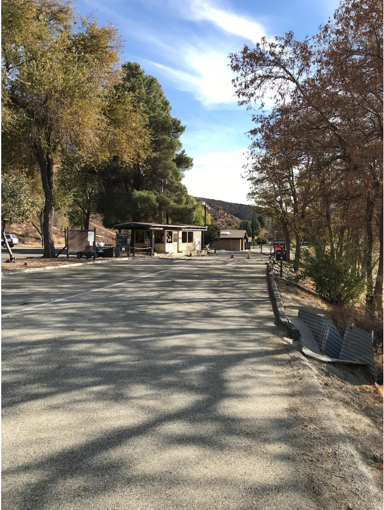
Building A3019K: Emigrant Landing Kiosk Building, Approx. 110sq. ft, built in 1975, and photo take from North West corner
