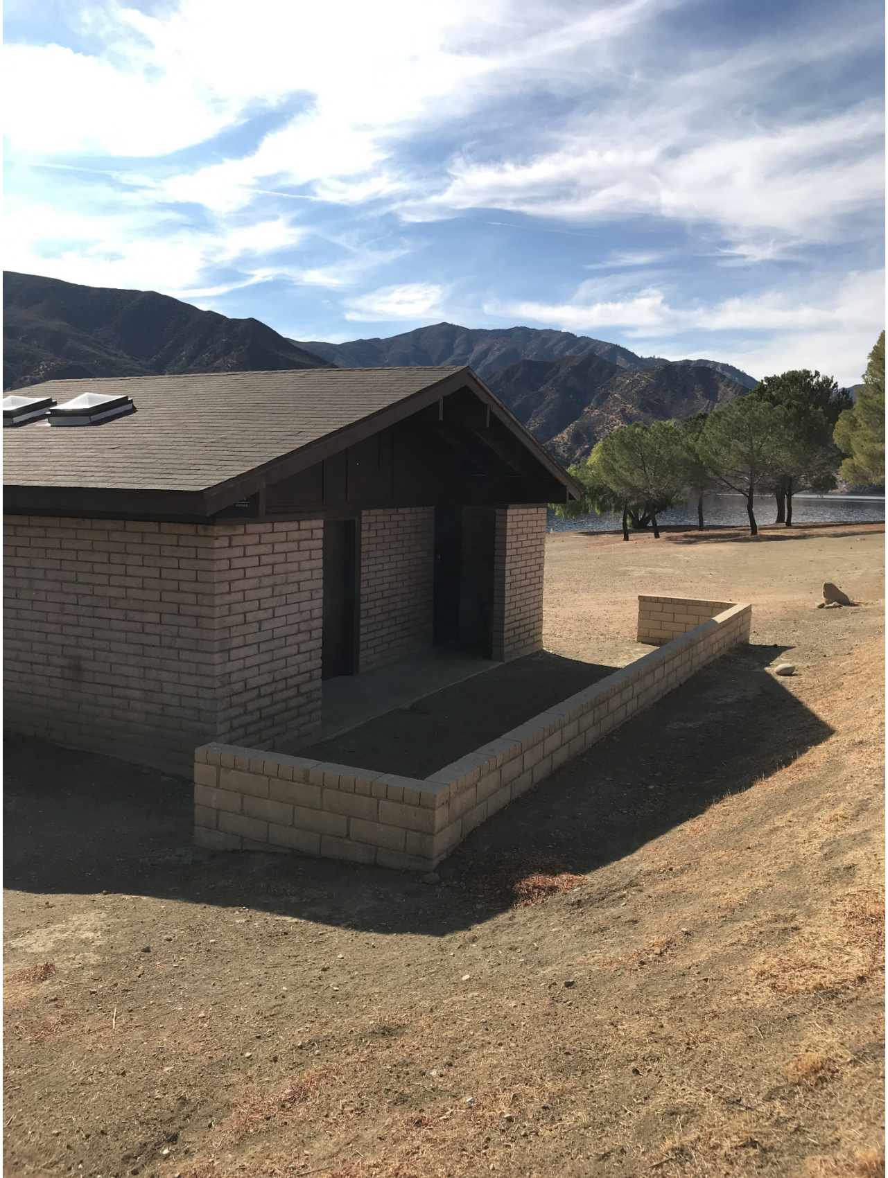
A3014R Spanish Point Restroom Service Basic National Forest (FS) 540 1973
