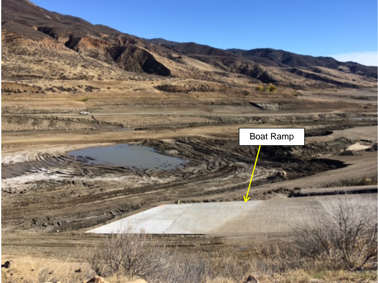
Figure 5. Extended boat ramp into Elderberry Forebay
