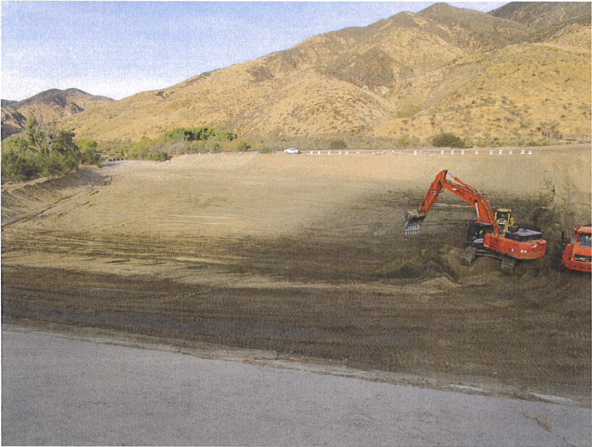
Figure 5. Castaic Creek Basin 1 sediment removal near completion (facing west)
