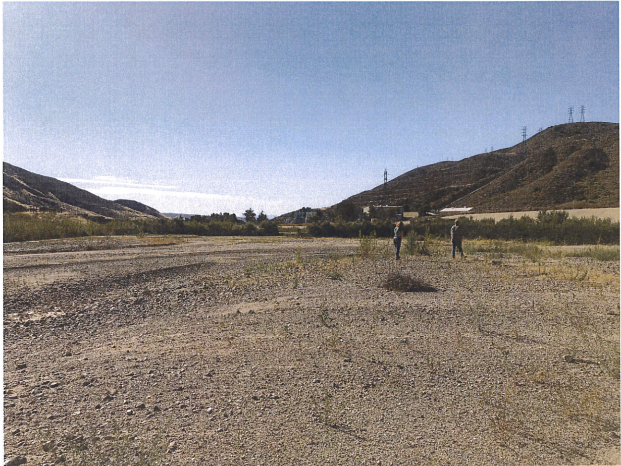
Figure 2. Castaic Basin 1 Pre-maintenance work (facing south)
