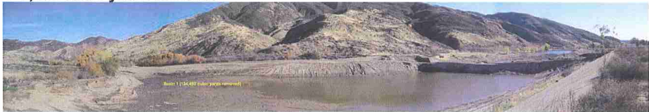
Post Construction Basin 1 134,450 cubic yards removed
