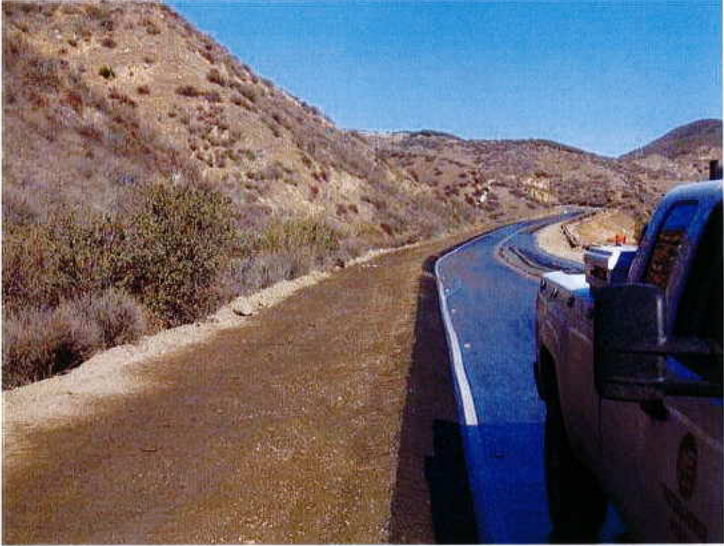
Looking north after fill
