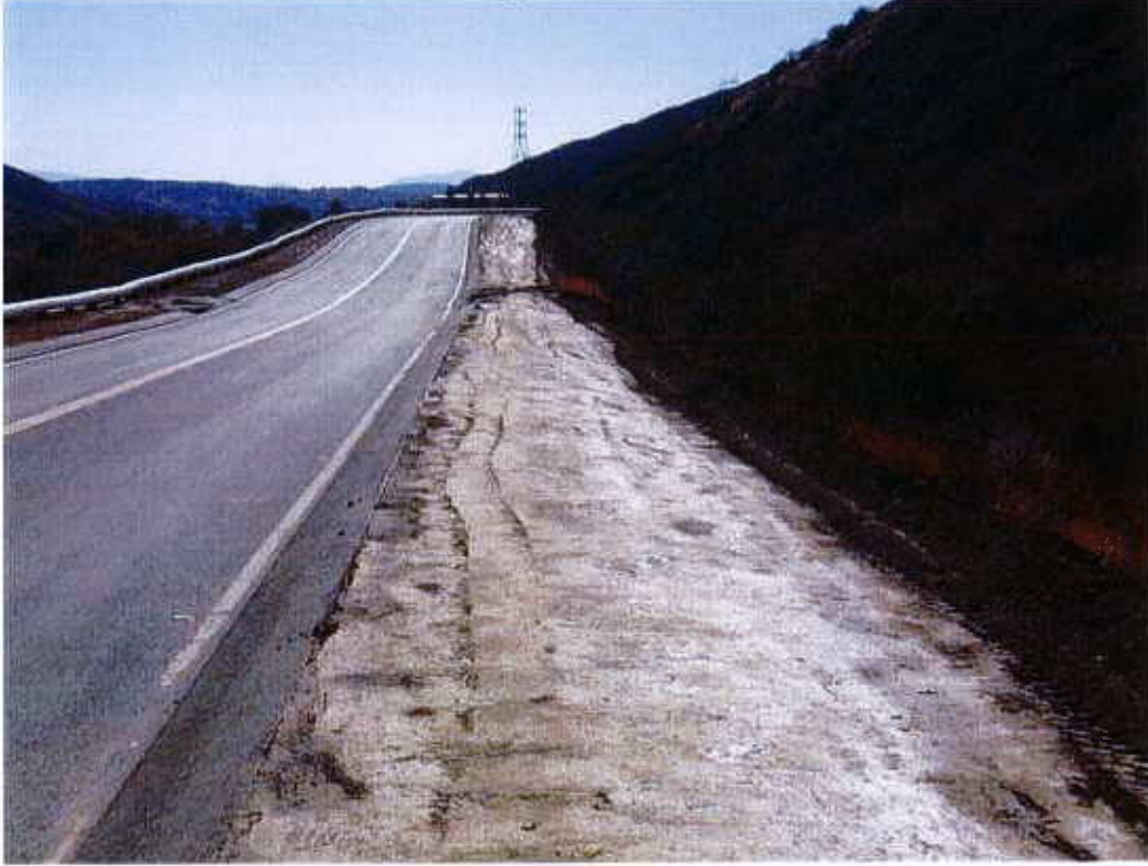
Looking south after fill
