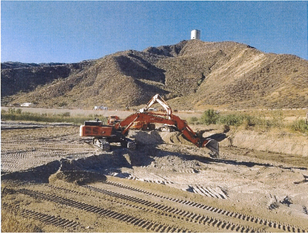
Figure 4. Castaic Creek Basin 1 during beginning of sediment removal (facing west)
