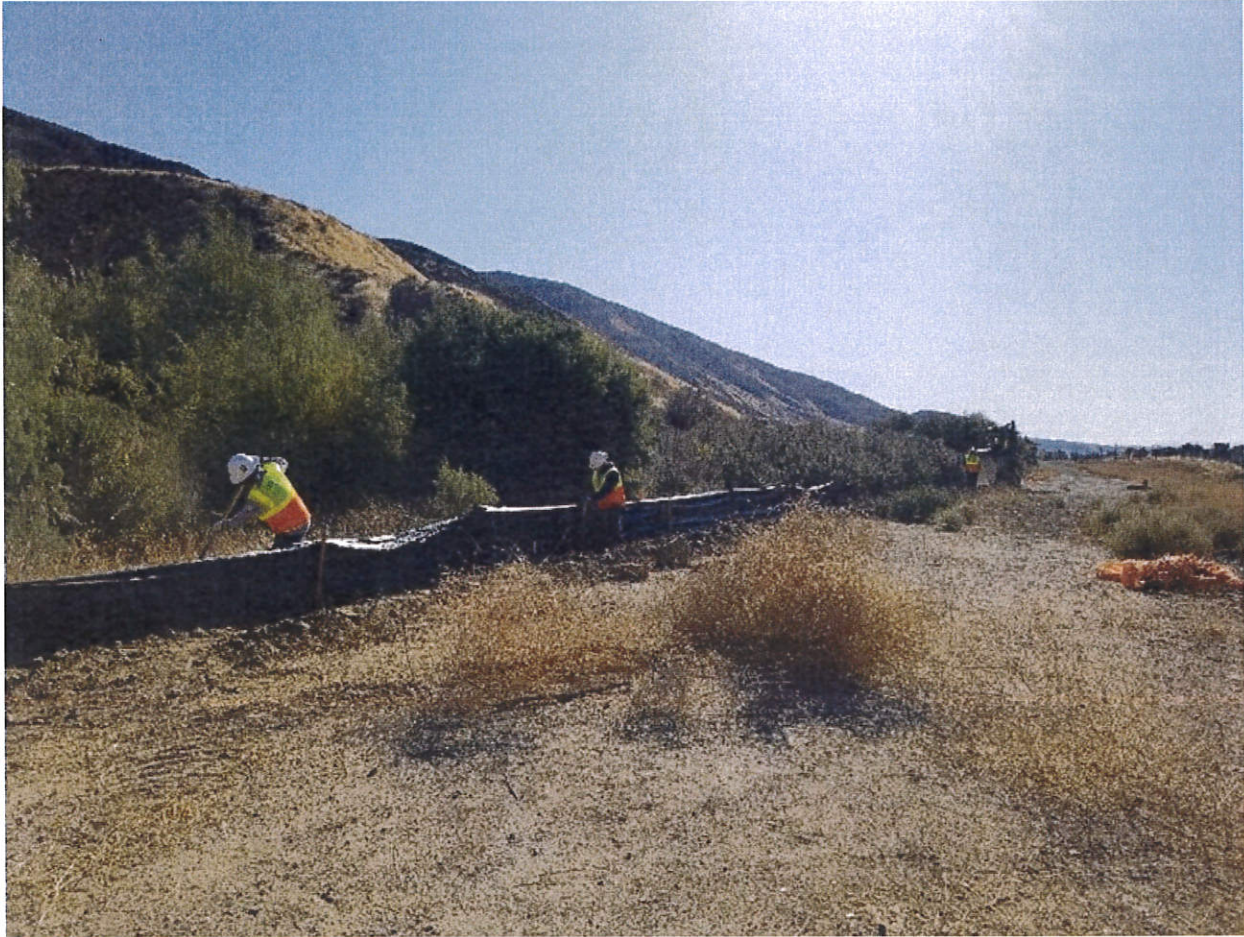
Figure 3. Castaic Creek Exclusionary Fence Installation (facing south-east)
