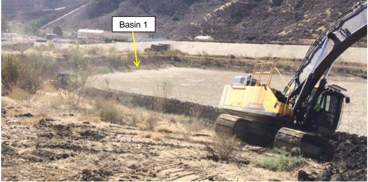
Figure 4. Castaic Creek Basin 1 during sediment removal (not yet completed)
