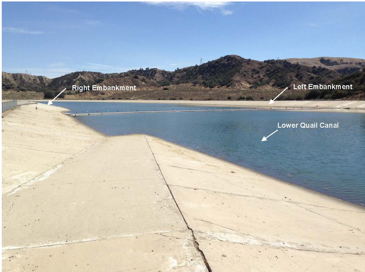
Figure 3.1-2. Lower Quail Canal Looking Downstream to Upstream
