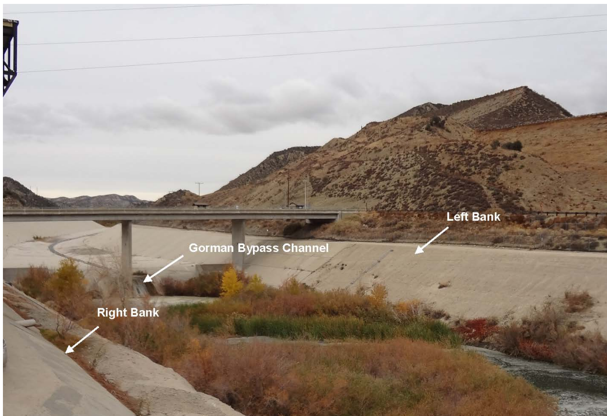
Figure 3.1-4. Gorman Bypass Channel Looking Upstream at Hardluck Road Crossing
