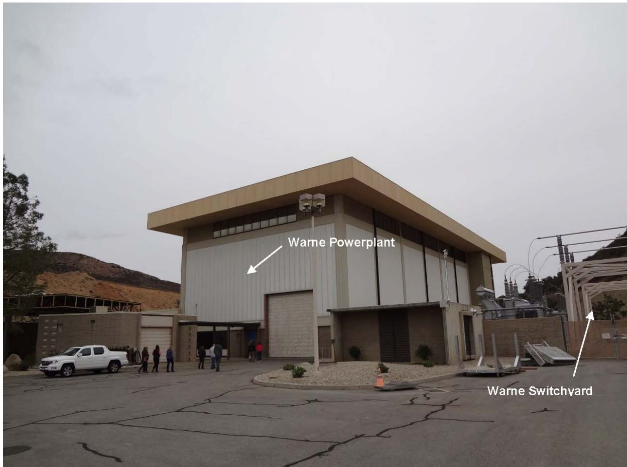
Figure 3.1-5. Warne Powerplant and Switchyard
