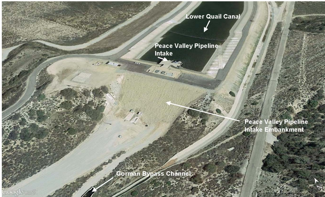
Figure 3.1-3. Peace Valley Pipeline Intake Embankment
